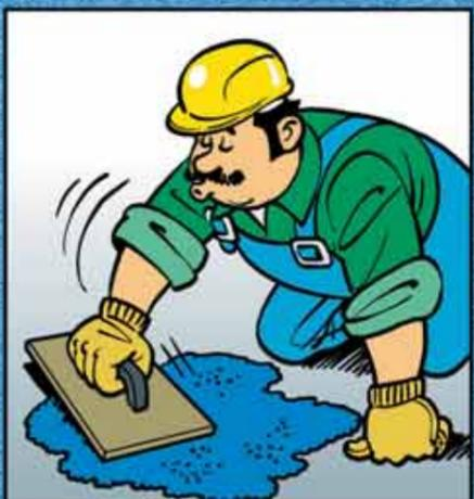
SI UNE COUCHE DE REVÊTEMENT OU DE PEINTURE EST POSÉE SUR LE BÉTON DURCI, UTILISEZ UN CURING COMPOUND SPÉCIAL.
