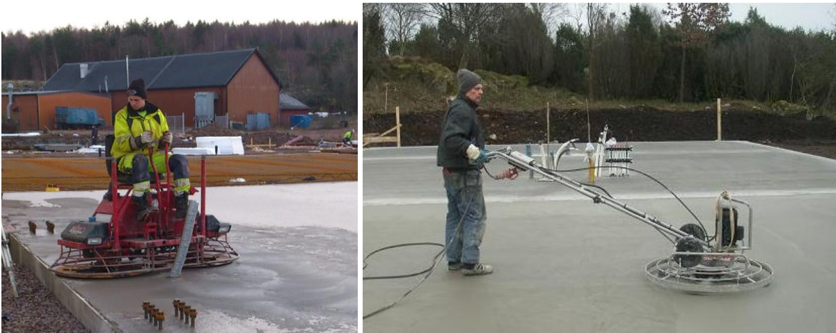
Figure 5. Surface trowelling at controlled age after casting
